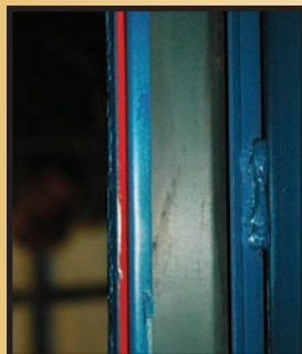
Apply red silicone to Retainer Strips to prevent leakage
