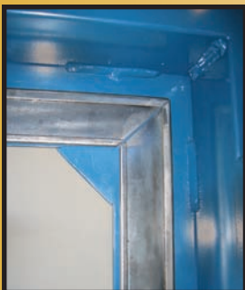
Plug-weld mild steel Backing Retainer Strips to existing Dryer door frame
