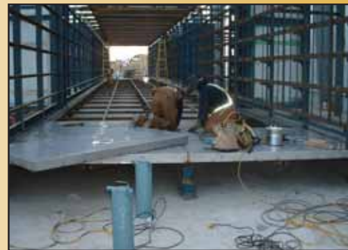
Above: Field installation of seal-welded floor panels
