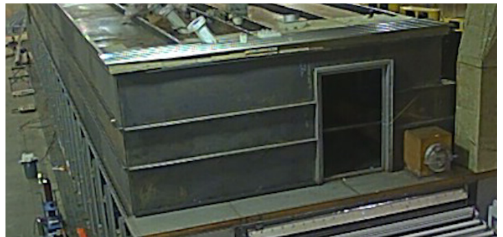
Seal-welded inner cladding
