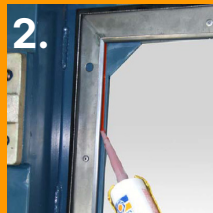
2. Apply red silicone under backing plate
