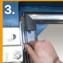
3. Insert stainless steel seal & corner seal
