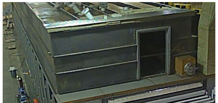
Seal-welded inner cladding
