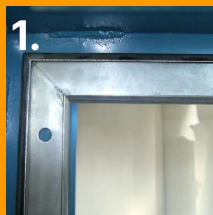
1. Mount backing plate
