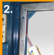
2. Apply red silicone under backing plate
