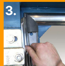
3. Insert stainless steel seal & corner seal
