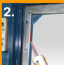
Apply red silicone under backing plate
