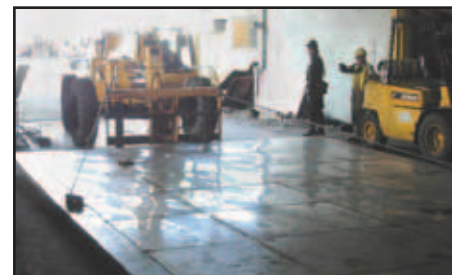
A stainless steel floor module is pushed into a dryer from the end.
