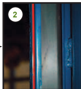
Apply red silicone under backing plate
