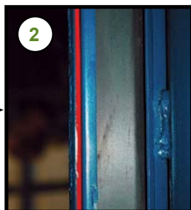
Apply red silicone under backing plate
