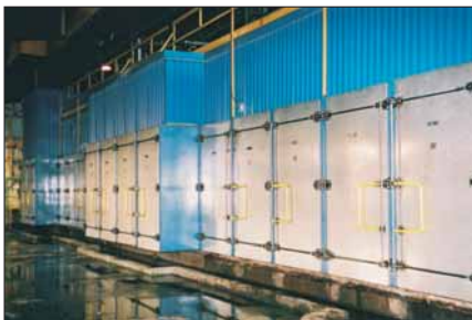
Westmill Two-Zone Rebuild
