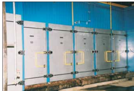
Westmill Doors and Side Panels - After
