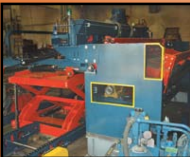
Installed scissor lift
