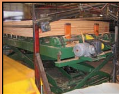
Powered top hoist installed to existing Dryer infeed
