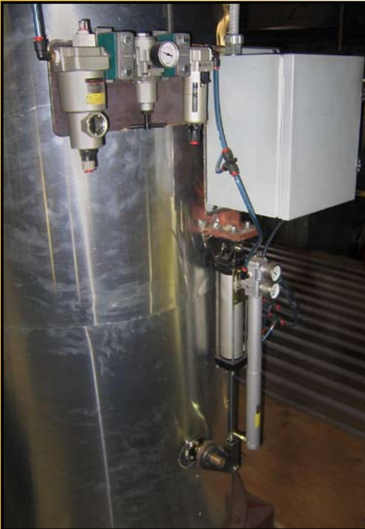
Westmill's Electro-Pneumatic Exhaust Stack Damper.
