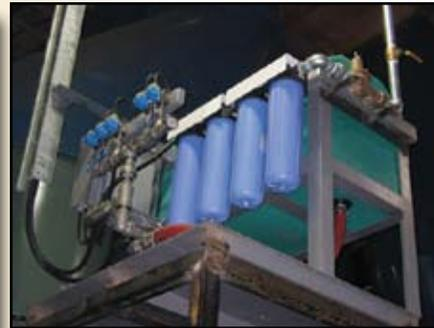
Above, Upper Duct Misting System tank and valves. Right, the Vaisala dewpoint transmitter. Below, the Dryer touch-screen image.
