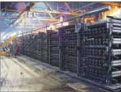
New floor under Weldwood's steam Dryer
